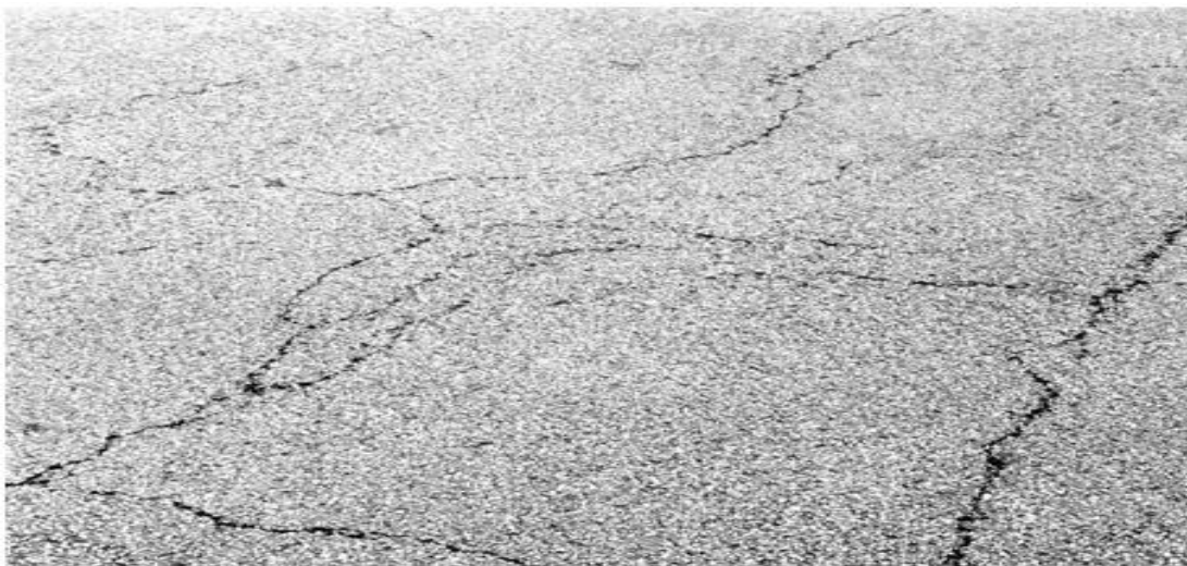
Figure 4. Block cracks Deterioration (Bukhari & Aman, 2023)
