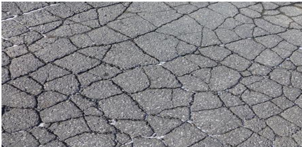
Figure 5. Shows Fatigue cracks and Deterioration (Ahmad & Khawaja, 2018)
