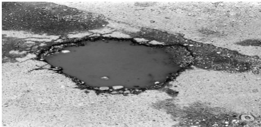
Figure 2. Potholes deterioration (Ahmad & Khawaja, 2018).
